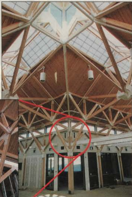
Angles, elevations complicated the exposed sprinkler piping. To cope, the sprinkler subcontractor had put the piping layout on a CAD file. Still, the job, with almost no standard fittings, was even more labor intensive than anticipated. Piping comes through column, runs along angled member.
