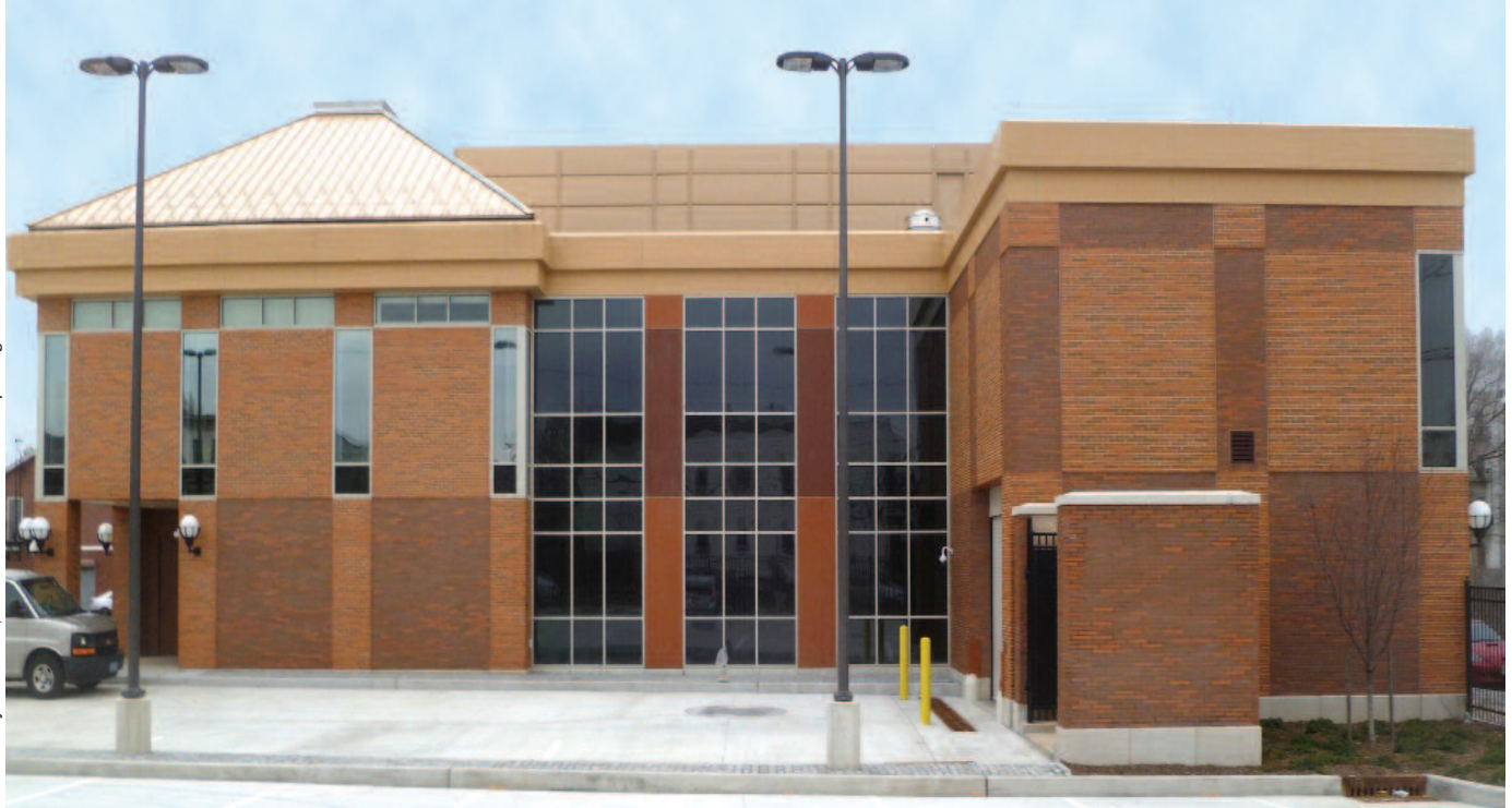
Locating windows at regular intervals achieves a fresh panelized look while still taking advantage of the durability of masonry.
